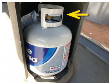
Find valve at top of tank
